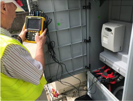
Fig. 5 Upstream inspection point of the charging station: The currents, on the board of the electricity meter's LV panel and the voltages on the respective LV busbars in the directly adjacent protective panel
