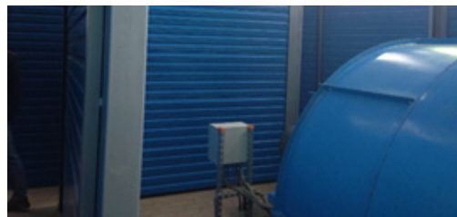
Fig. 9 Real Noise Measurements in Work Environment
